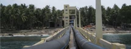
Low-temperature thermal desalination water plant set up in Lakshadweep islands by MoES converts seawater to potable water for islanders
