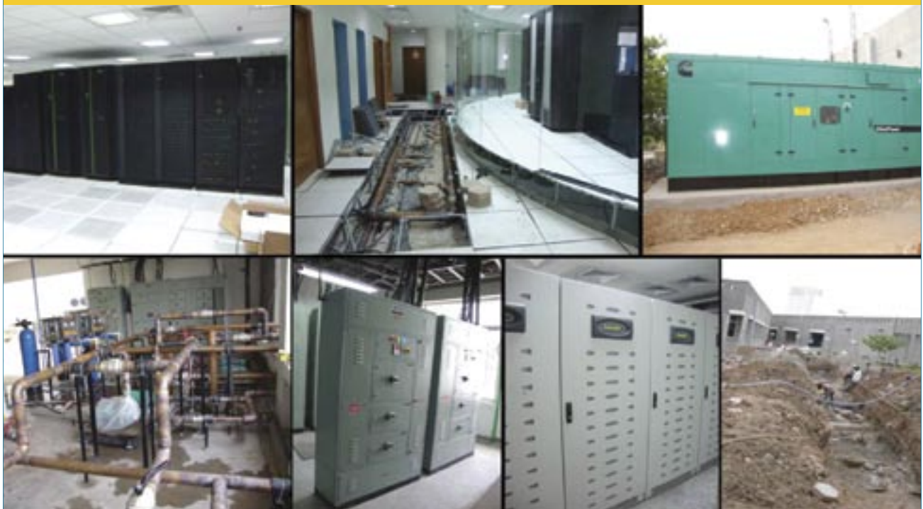
Fig. 3.2: HPC and Technical Facilities
