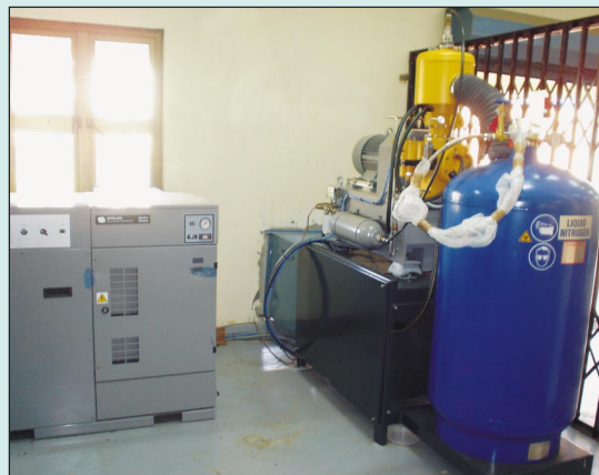
Liquid Nitrogen Plant at NCAOR
