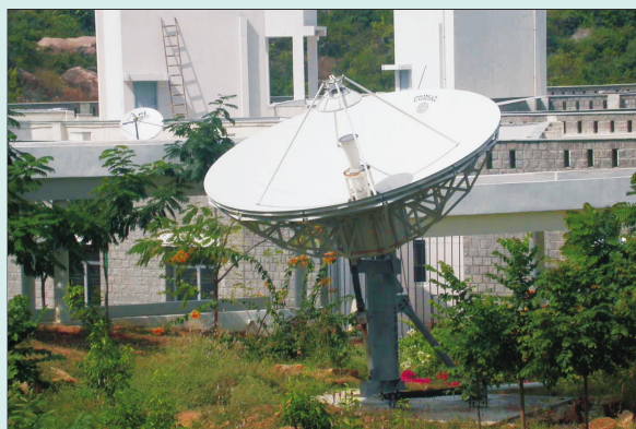
VSAT Terminal with 4.5 m Antenna established at INCOIS.
