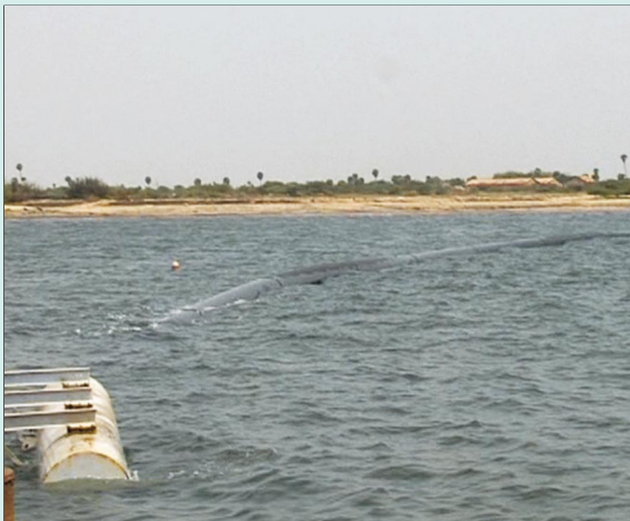
Towing of 1 m dia 700 m length HDPE pipe.
