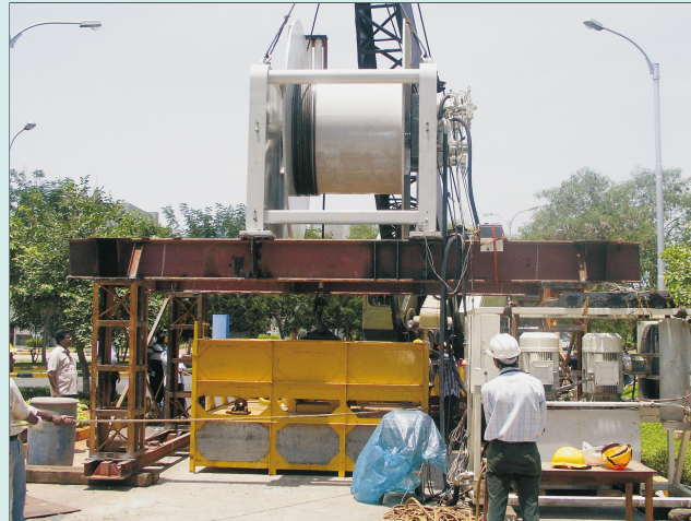
Winch Load Test in progress.
